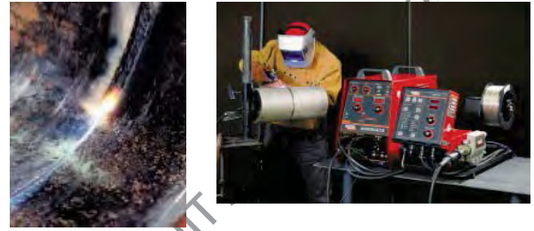
STT process using 100% CO 2 and .045 in. wire. Inside of an 8 in. x .375 in. wall API 5L-X52 pipe, welded in 5G position.
